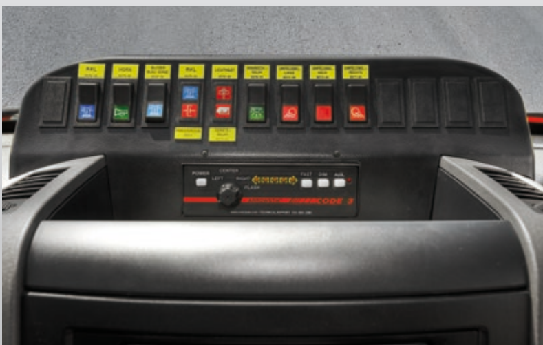
Switch console in the control panel
